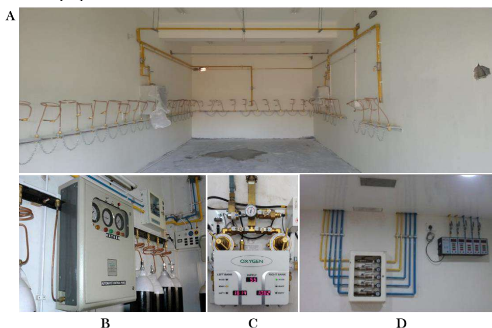
Figure 3.5: (A) Manifold room. (B) Oxygen manifold control panel (analog). (C) Oxygen manifold control panel (digital). (D) Manifold alarm system and isolation valves
